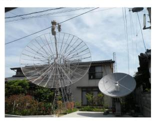
JA4BLC has two dishes (dish brothers) for use on L to K-band; L and S-band are on the 6 m dish, and an X band feed on the 3 m dish.
